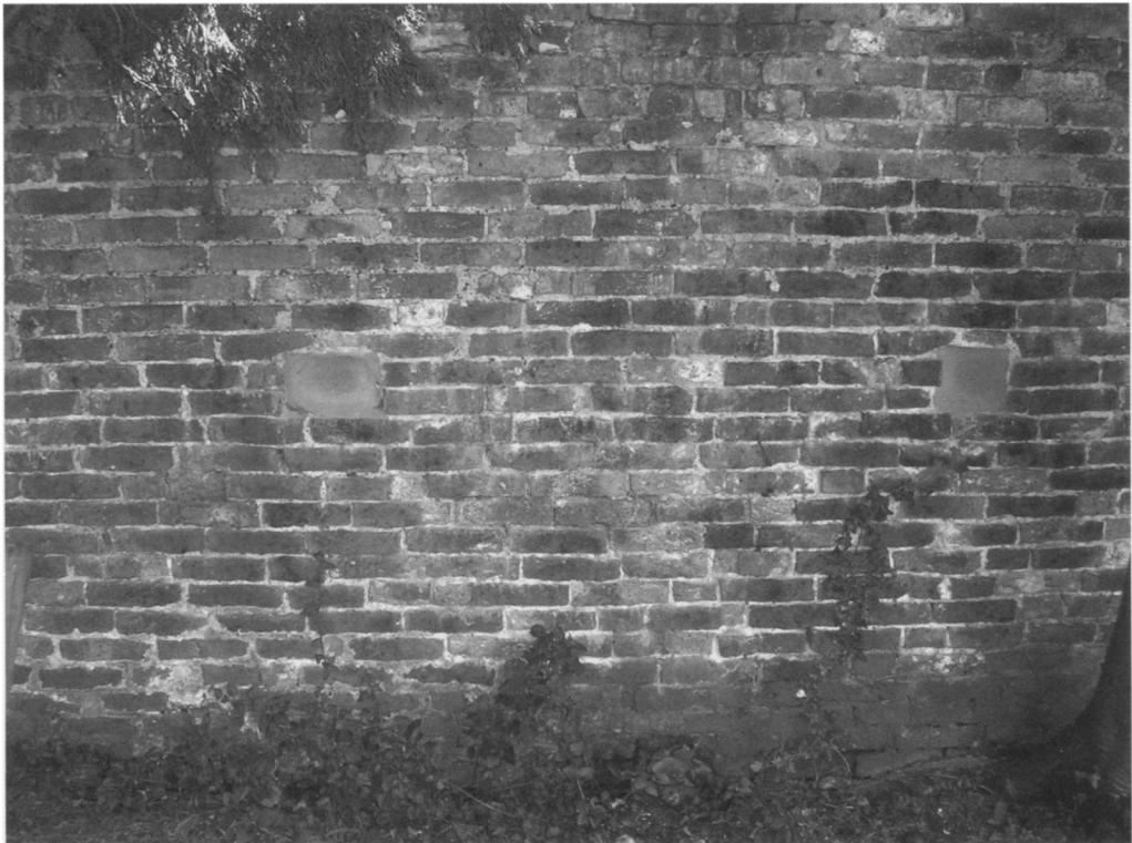
Figure 8. The garden sides of the walls at Thrybergh have been lined with brick to retain heat. They appear to be connected at the bottom only – where at a height of about 3 foot and distance of about every 5–6 foot, stones have been cut to the dimensions of the brick – and effectively link the stone outside to the brick inside of the wall. Photo: Jan Woudstra
