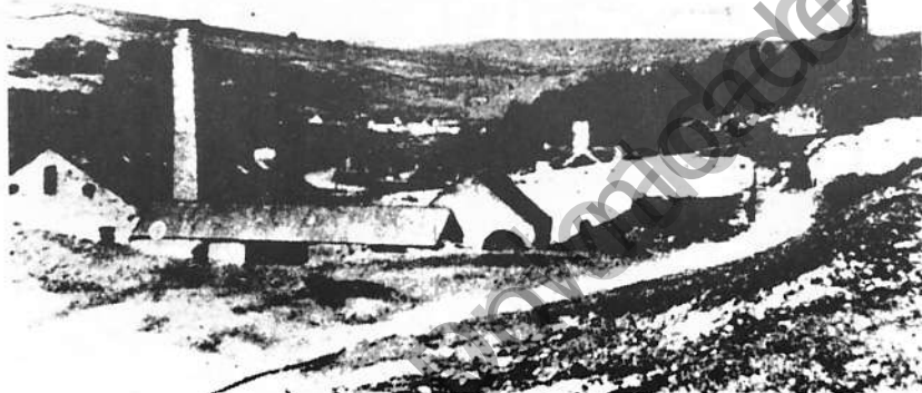
Plate 7. The Nenthead smelt mill in about 1910. The tower to the right was above the Brewery Shaft and gave an extra head of water to the hydraulic compressors (Richardson Coll.)
