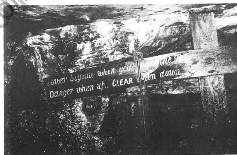
Plate 15. Signalling system at the foot of an incline in Caplecleugh Low Level:- "Lower Signal when you get to the Top. Danger when up, CLEAR when down". Sept. 1982 (M.F.Critchley)
