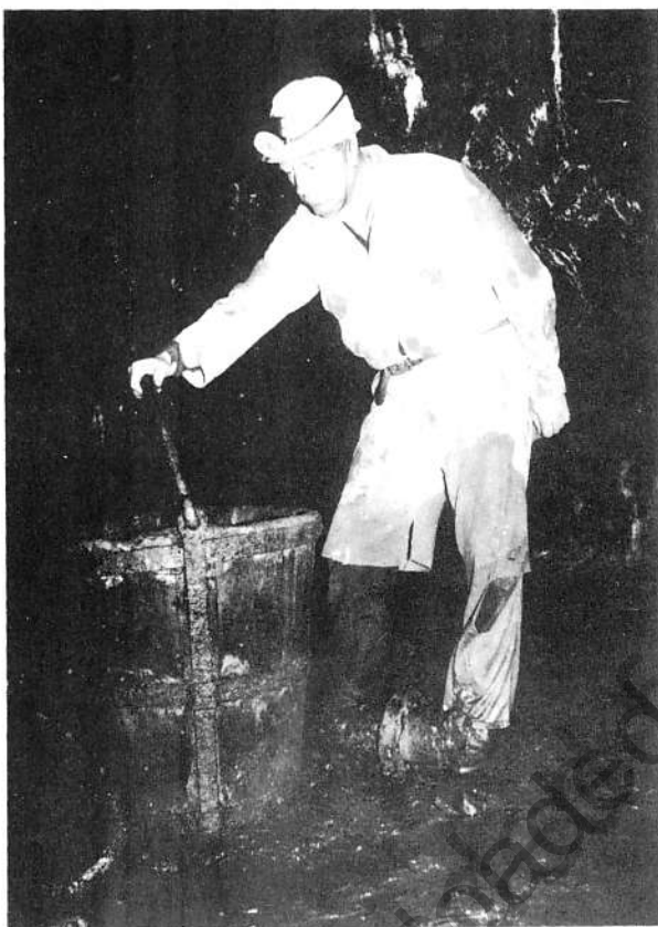
Plate 16. Kibble and 'old man' at the Engine Shaft in Rampgill Mine, Sept. 1980 (M.F.Critchley)
